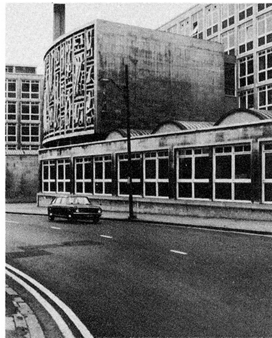
Fig. 2 Modern exterior of Mechanical Engineering Building at Leeds
